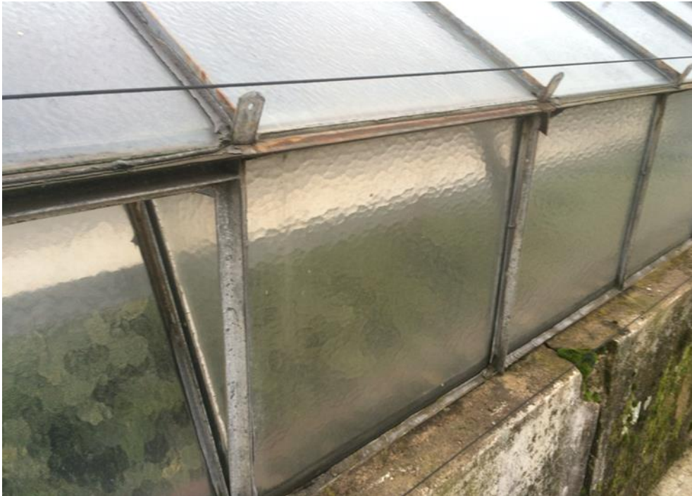
Figure 3.5. A greenhouse in France glazed with textured glass to achieve diffusion.
